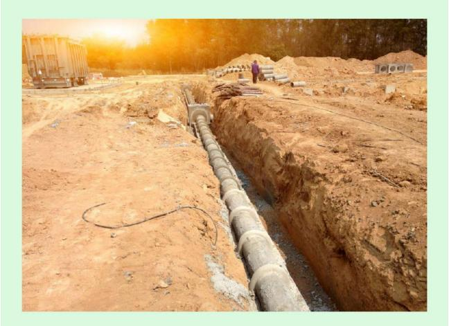
Concrete drainage pipe is laid along the roadside.
