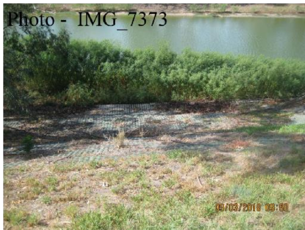
Ch. 4050 – Reno Mattress at River Side Toe
