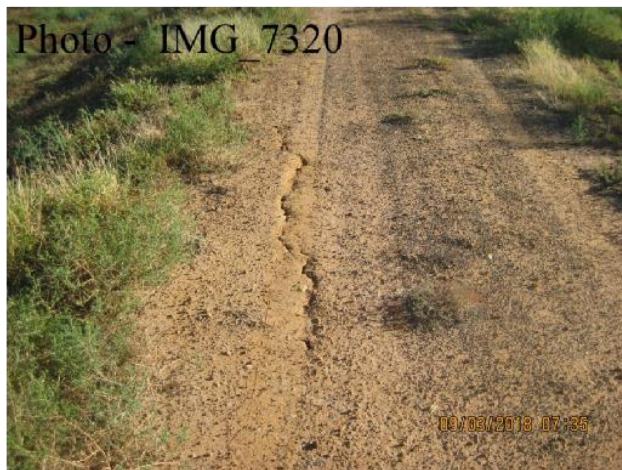
Ch. 7950 – Crack River Side of Crest
