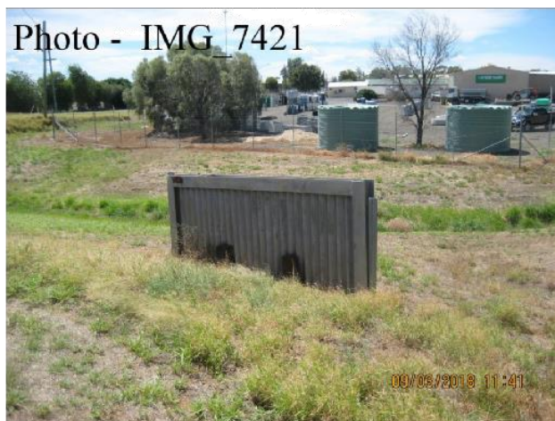
Ch. 6700 – Flood Gate for Western Rail Crossing
