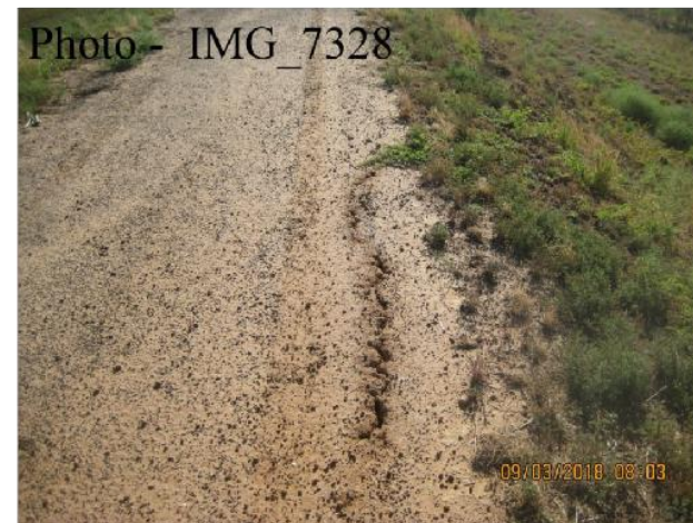
Ch 50.- Crack Town Side of Crest
