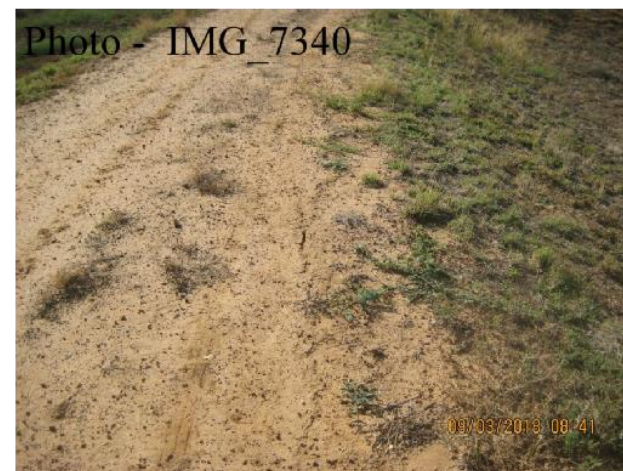
Ch. 1600 – Crack Town Side of Crest
