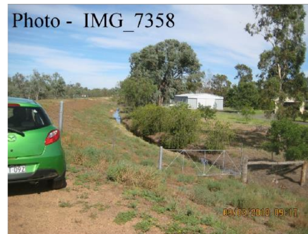
Ch 2900 – Ponding Water at Town Side Toe
