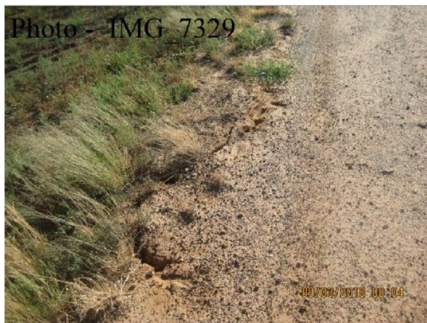
Ch. 50 – Crack River Side of Crest
