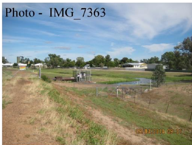
Ch. 3400 – Ponding Water at Town Side Toe
