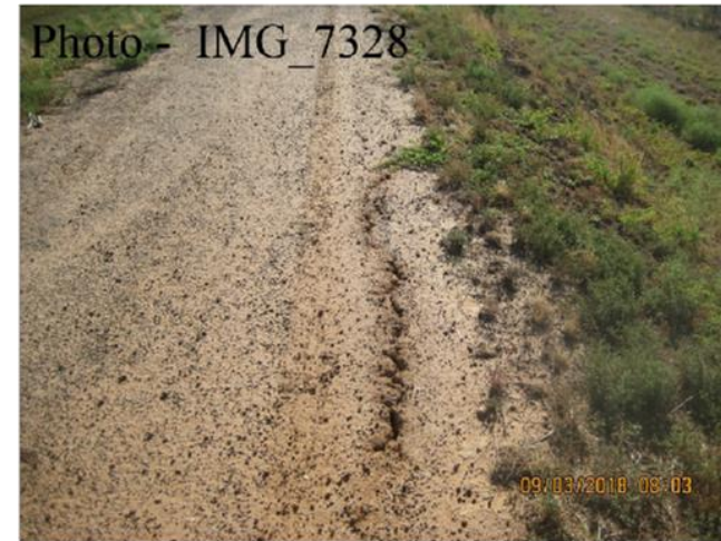
Ch 50.- Crack Town Side of Crest
