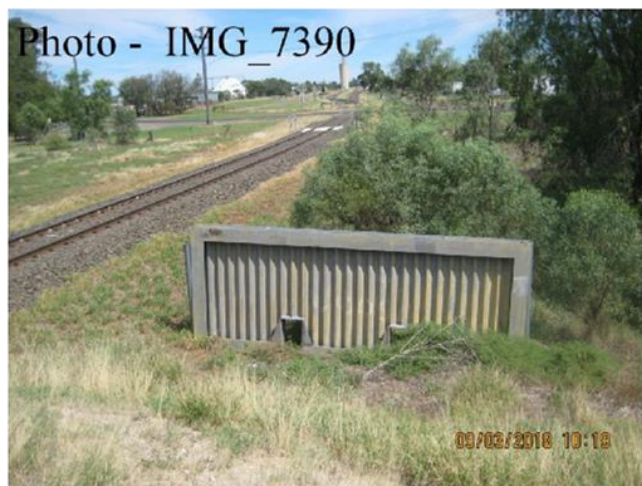
Ch. 4700– Flood Gate for Eastern Rail Crossing
