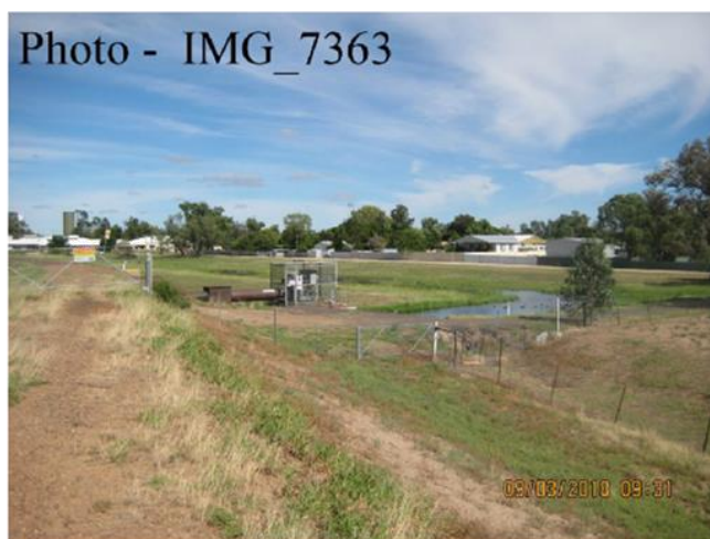
Ch. 3400 – Ponding Water at Town Side Toe
