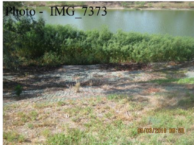
Ch. 4050 – Reno Mattress at River Side Toe
