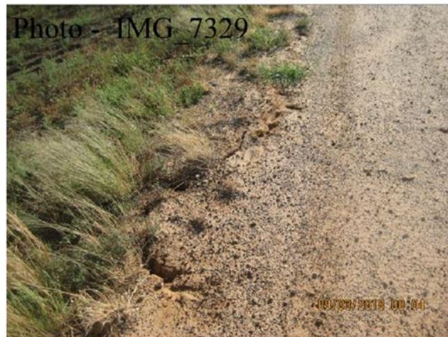
Ch. 50 – Crack River Side of Crest
