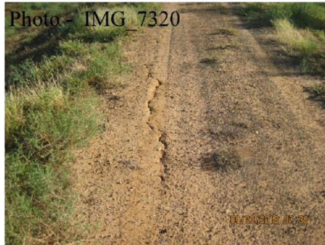
Ch. 7950 – Crack River Side of Crest
