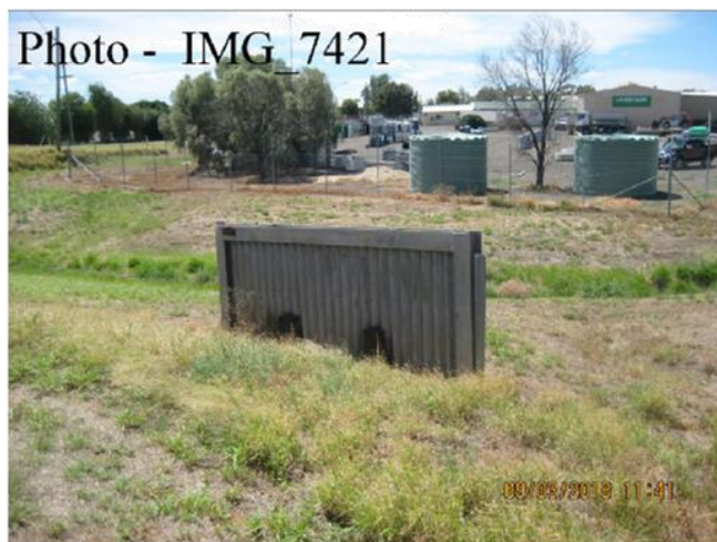
Ch. 6700 – Flood Gate for Western Rail Crossing
