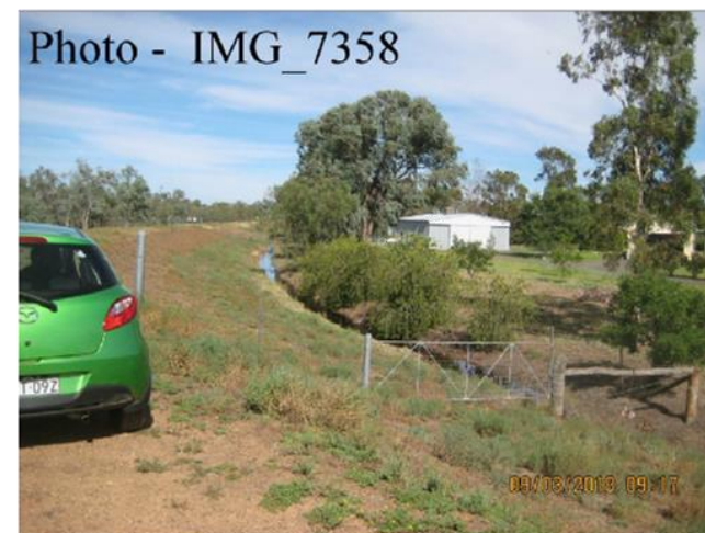
Ch 2900 – Ponding Water at Town Side Toe
